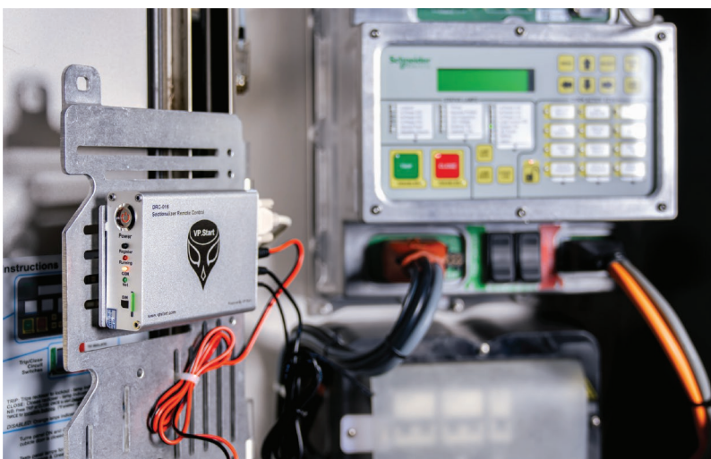
▲ DRC-018 Remote Control With Sectionalizer
