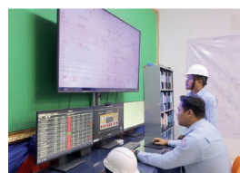
Electricity of Siem Reap
